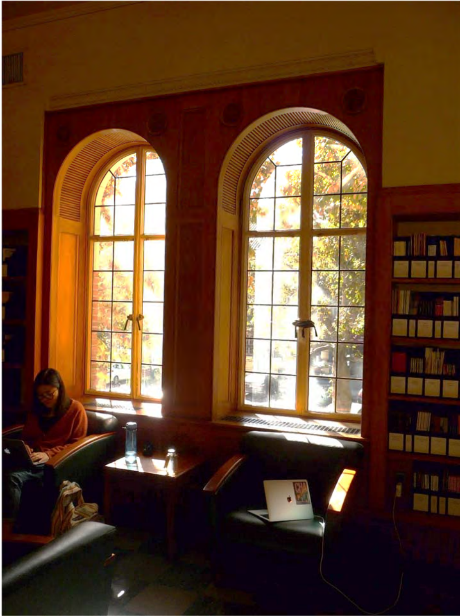
Paired arched window openings with decorative sycamore wood surround, steel casement windows
