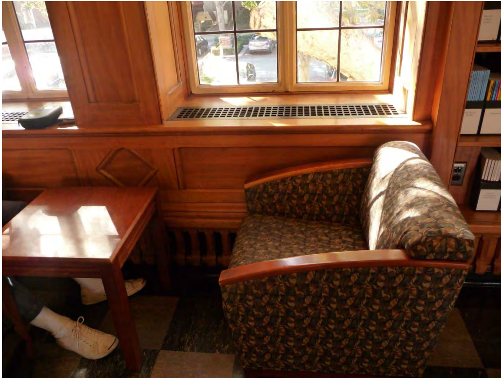
Window sills with bronze grilles and wood paneling and grilles beneath
